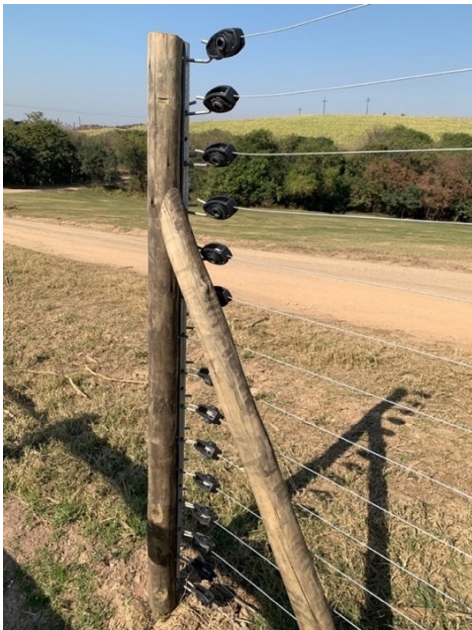
1.5m high electric fence
