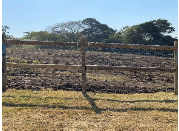
Combination of timber paddock fencing and welded galvanized mesh yard fencing
