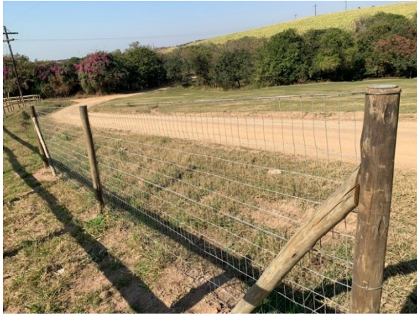
Combination of timber paddock fencing and welded galvanized mesh yard fencing
