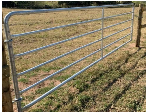
Galvanized steel gate
